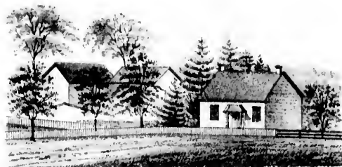
FARM RESIDENCE OF DAVID SIXSMITH ESQ. RICHMOND TOWNSHIP ONTARIO.
